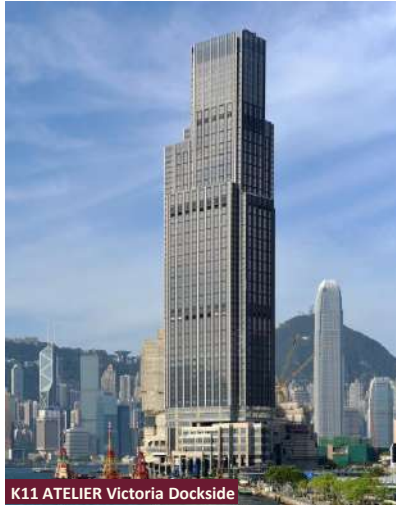
K11 ATELIER Victoria Dockside
